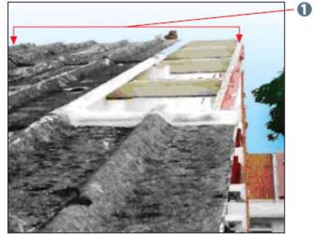
1. Roof tiles removed
